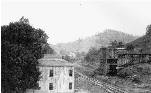
Train tracks with one line running beneath a coal tippie, Ely area of Knox County, early 1900s. Photograph courtesy of the Michael C. Mills Photographic Archives of the Alice Lloyd College McGaw Library, Pippa Passes, Kentucky (negative number 75C-LL45-78).
